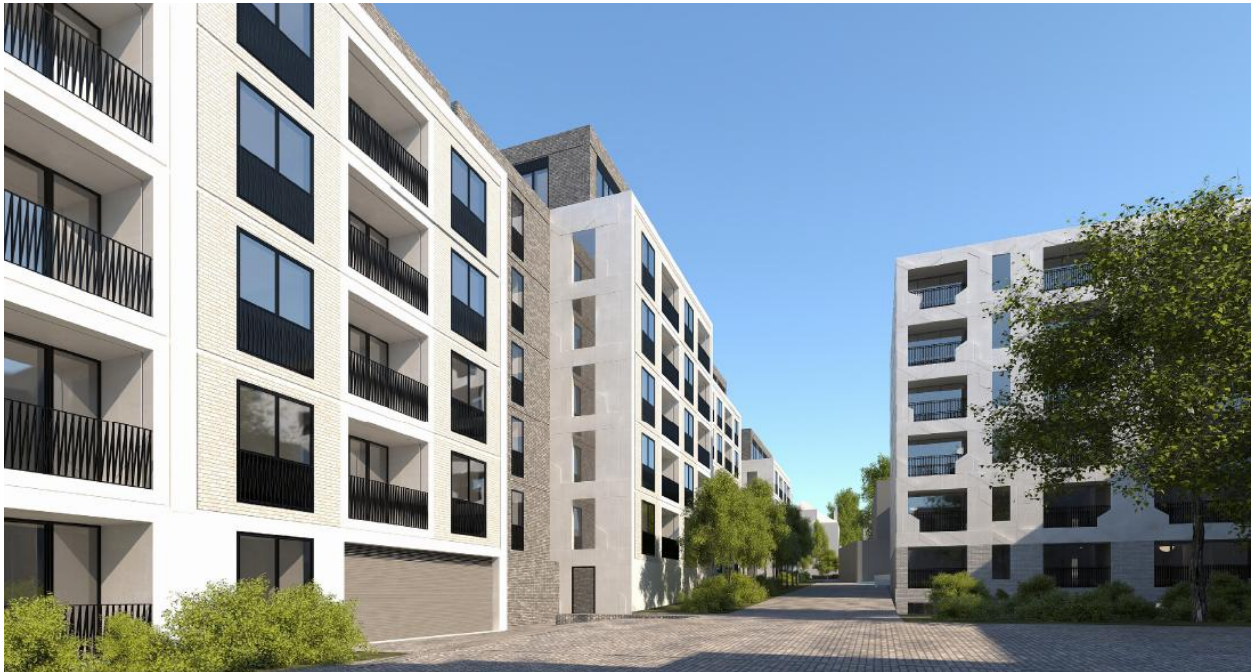
Image 1.12 - Looking south from Weston Park access. (Source Applicant)
